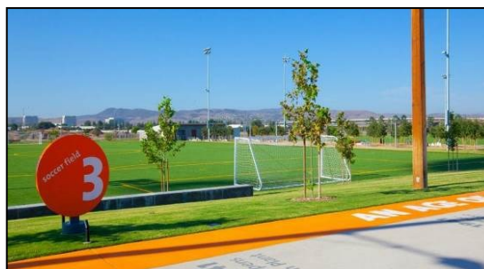
The Orange County Great Park (OCGP) is a large, partially developed regional park with recreation facilities to support the arts, gardening and agriculture, sports and fitness, events and festivals. This park will continue to be developed according to its approved master plan.
