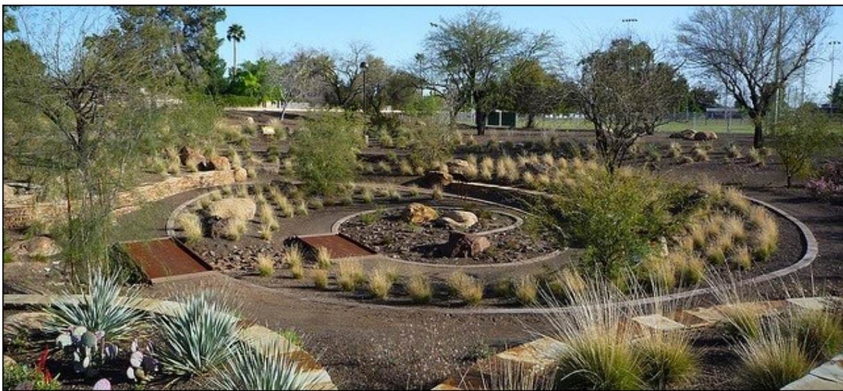
Spiral garden with infiltrating stormwater element, Chaparral Park, Scottsdale, AZ
