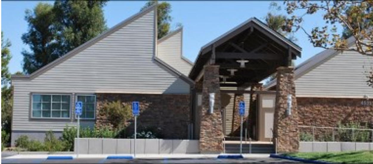
Northwood Community Center underwent a modernization and expansion in 2013
