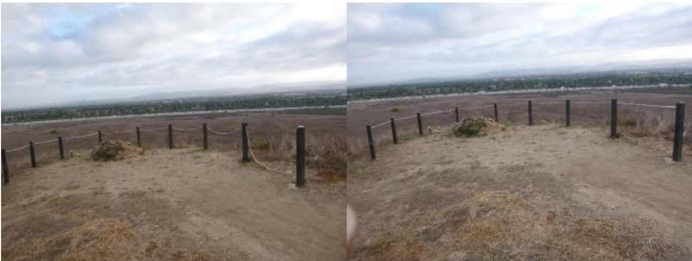
Vista Point Post and Rope Fence Repair
