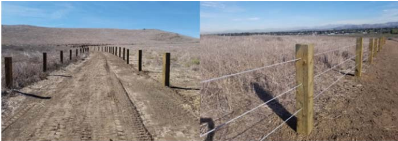
Quail Hill Trail South Fencing Installation
