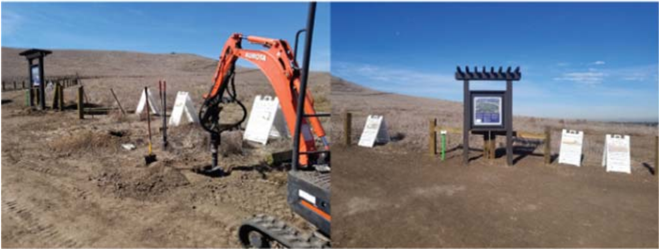
Quail Hill Trail South Fencing Installation
