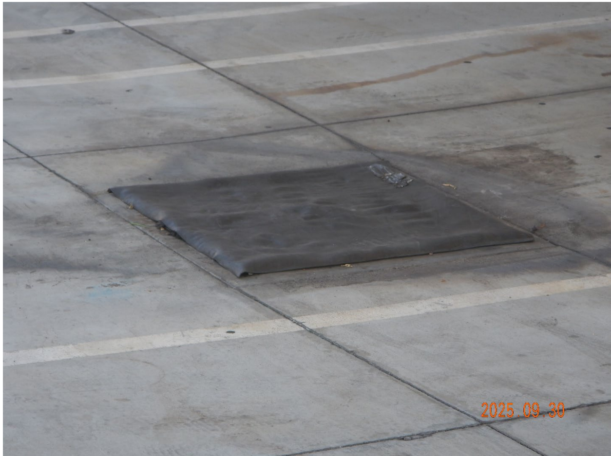
Close-up of the inlet cover at the front northern loading bay.
