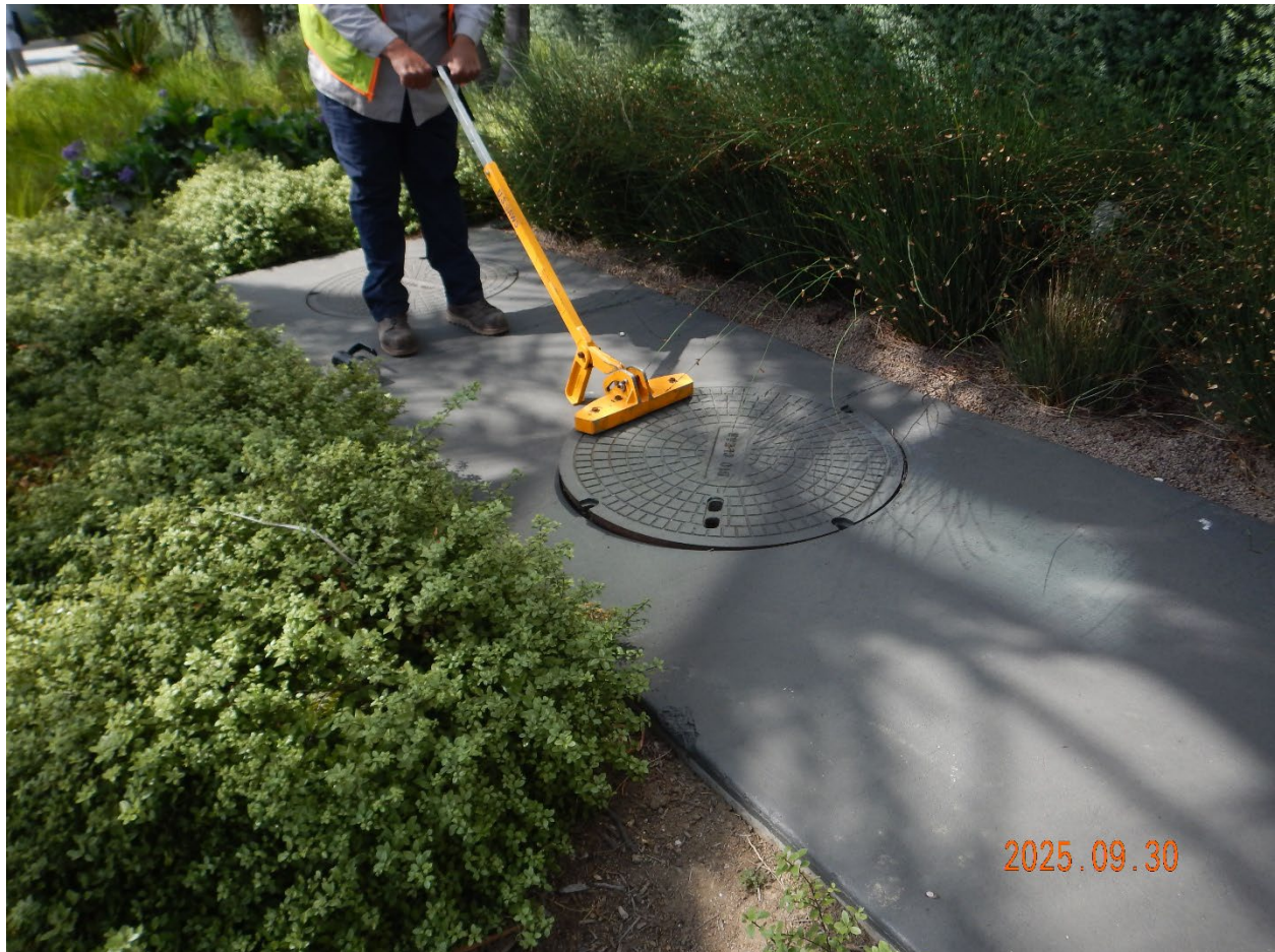
A City field inspector removed the lid to the chamber containing pre-filter cartridges for the biotreatment system. The nearby vegetation appears healthy despite dry topsoil.
