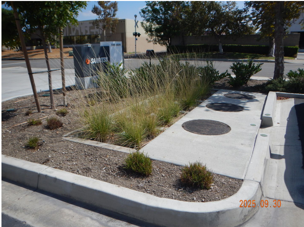
View of the site's BioClean Modular Wetlands Linear System, specified in the WQMP, is shown with mildly distressed vegetation.
