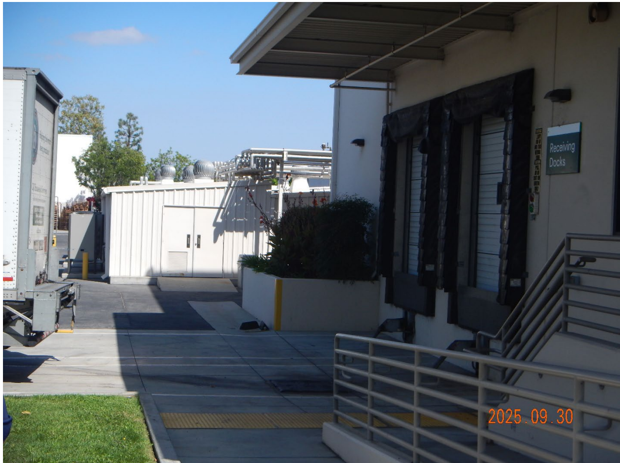
View of the front northern loading bay. The site's representative states that a rubber cover seals the storm inlet to keep automotive fluid from entering the drain.
