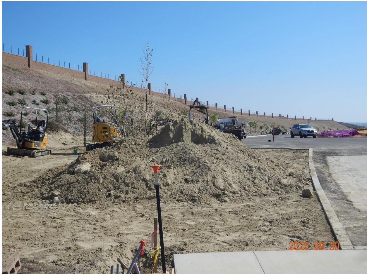
The photo shows soil excavated for utility installation.
