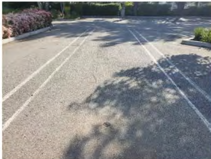
Photograph 14: Typical view of patched asphalt that was cored during the performance of the Phase II ESA for the subject property. This is one of 12 cored locations on the subject property.
