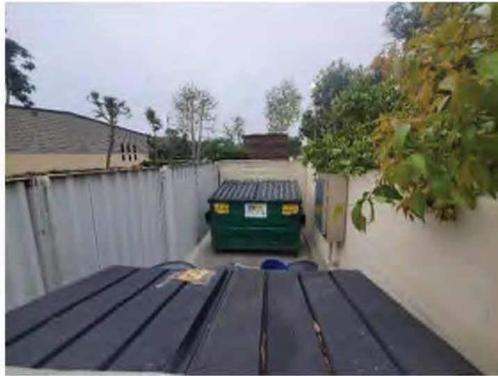
Photograph 13: View of interior of trash enclosure that adjoins the site of the roll-off box. The enclosure contains dumpsters for the disposal of site waste.
