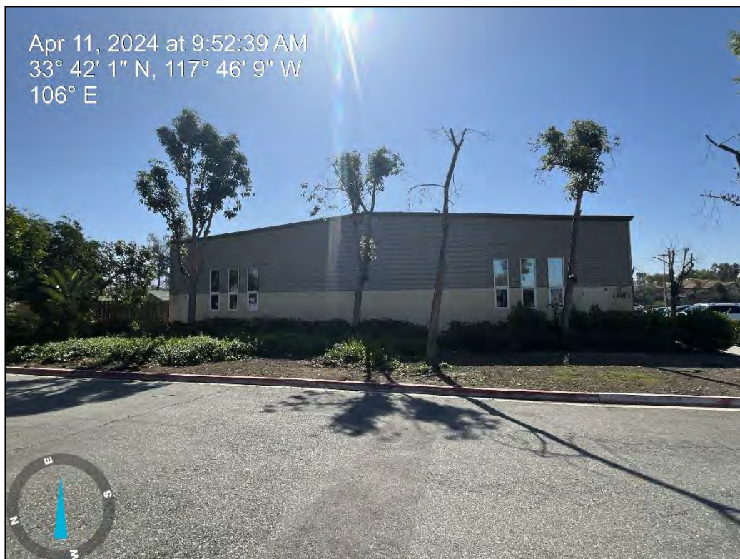
Looking east at the main church building.
