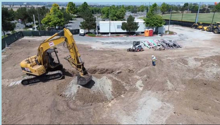
Underground demolition completed
