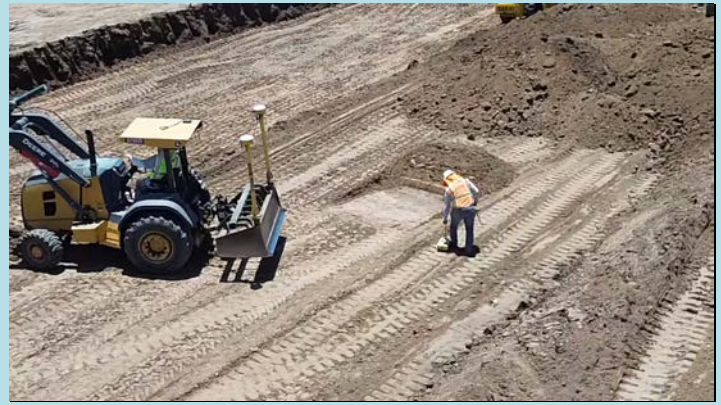
N & M geotechnical inspector verifying compaction
