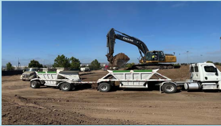
Excess dirt export underway
