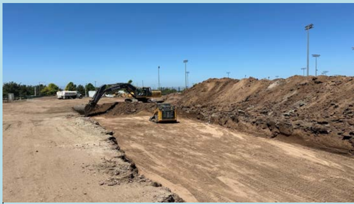
Over ex and compaction work ongoing for main building pad
