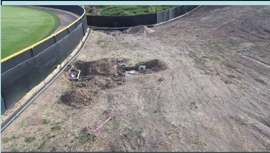
Completed high-line installation and confirmed operational
