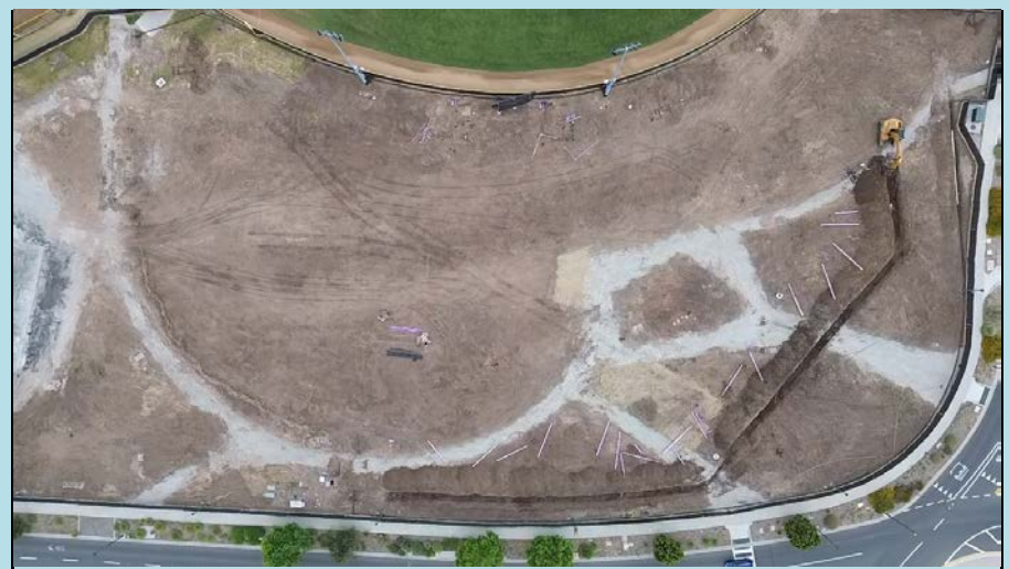
Aerial view of progress at job site
