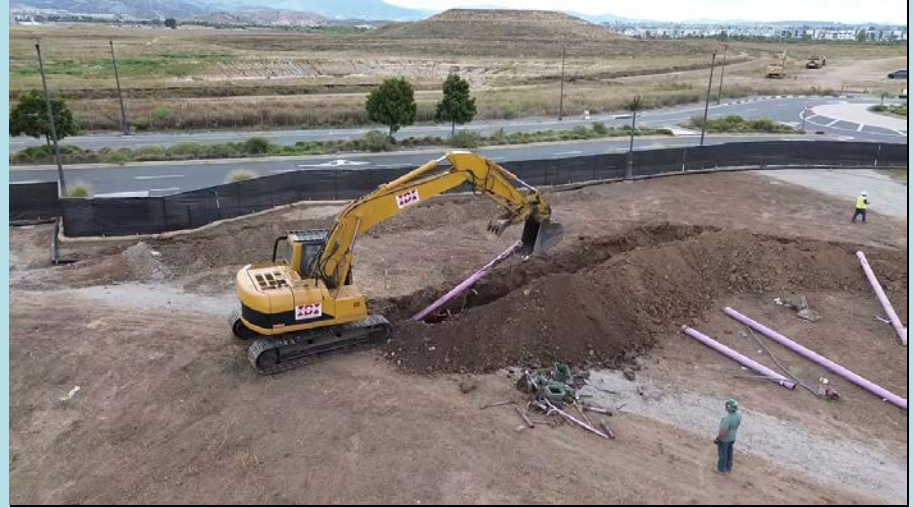
Underground demolition has commenced, irrigation lines being removed
